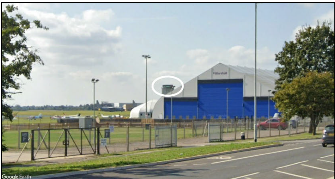
Figure 5 Ground-based view of the ATC Tower at Cambridge Airport (visual control room circled)
