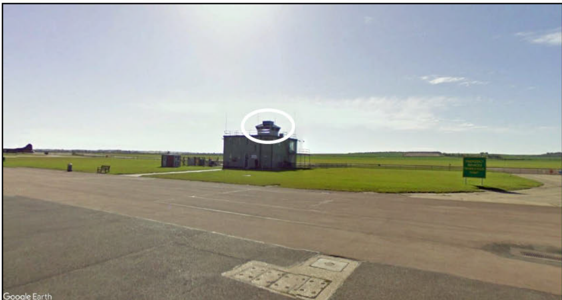
Figure 10 Ground-based view of the ATC Tower at Duxford Aerodrome (visual control room circled)
